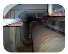
Ballast pipe on a 300mtr grain carrier had become so badly corroded the vessel was struggling to take on board ballast. Due to the confined space and restricted access the surfaces of the pipe could only be manually abraded. Once cleaned 302 Epoxy Repair Cement was applied to the repair surface. 301 Epoxy Resin and Hardener and Glass tape were applied once the repair paste had cured
