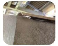
Leaking ammonia chemical line required sealing in an emergency. The surface of the pipe was mechanically abraded and a pre-formed steel plate bonded over the hole using 106 Metal Repair Paste XF. The repair was then overwrapped using 301 Epoxy Resin Hardener and Glass Tape
