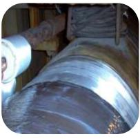
When used with 301 Epoxy Resin and Hardener 701/703 Glass Tape can be used to encapsulate isolated leaks or to encapsulate long lengths of large diameter pipe work.
